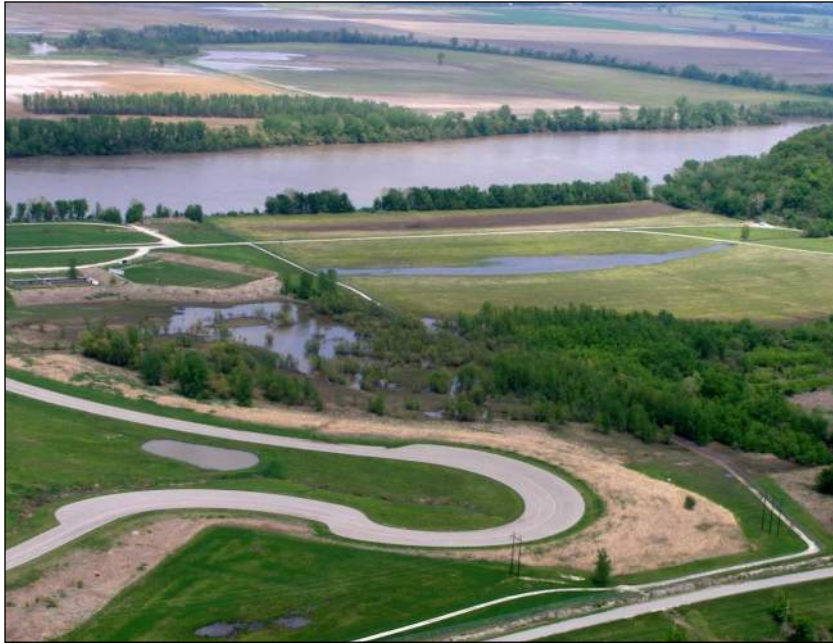
Figure 2.3—South Site Aerial
